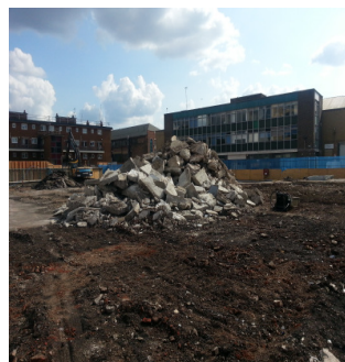
Concrete slab removal
