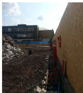
Canal wall hoardings
