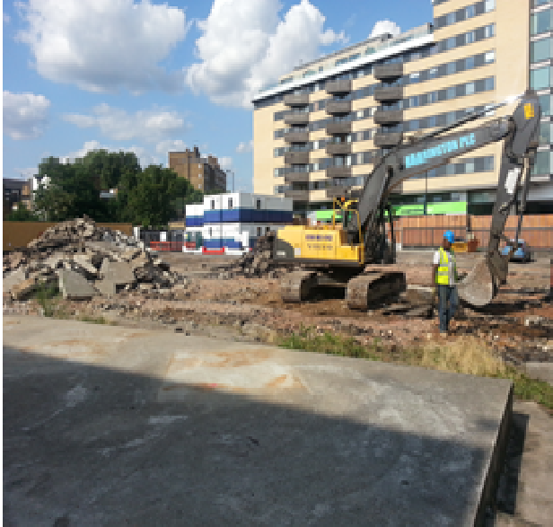
Break out of hard standings looking towards the North East elevation
